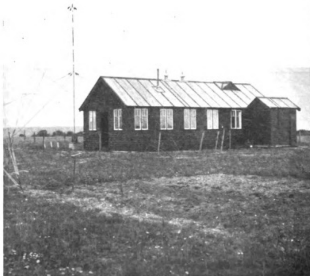
Transmitting Station at Southwold showing mast.
