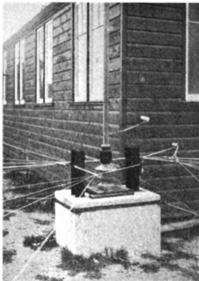
Base of insulated Transmitting Mast at Southwold.
